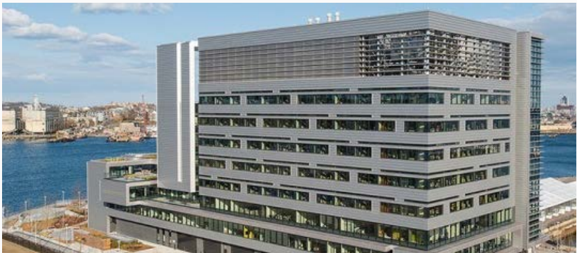
Spaulding Rehabilitation Hospital in Boston, designed by Perkins + Will and awarded LEED gold – you can see the mechanics on the top floor of the building
