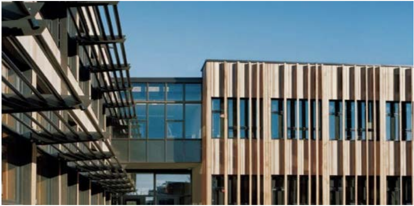
Sidwell Friends School, designed by KieranTimberlake, employs multiple solar shading devices throughout the facade, to block hot midday solar radiation
