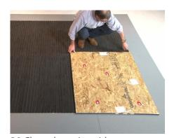
**20** Clean the unite with a vacuum. If construction is to continue in the building, protect the unit with plywood sheathing.
