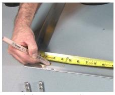
**12** Mark the center point location of the first two rails onto the frame using a carpenter's pencil.
