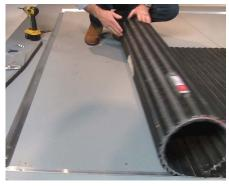
**8** If it appears that the overall grid section is too short, it may be necessary to stretch the section by rolling the mat back on itself.
