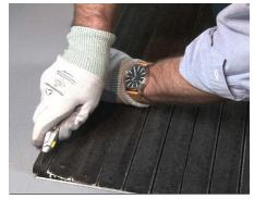
**10** For proper fit, the end trim can be cut in any of the grooves that are spaced 1/8" apart using a sharp utility knife. Score several times to cut completely through the material.
