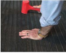
**7** Lightly tap across the connection with a rubber mallet to ensure the feet are seated in the connectors. Repeat this step for all remaining modules.
