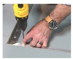
**15** Using 5/16" masonry drill bit, drill out both holes for the locator bar anchors to center the supplied locator bars on the lines marked on the floor.
