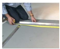
1 Start by dry fitting all frame pieces within the area and use a tape measure to ensure a proper fit. For odd-shaped layouts, match frame tags to the drawing on the pack list.
