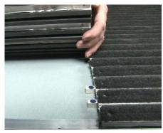
**17** At any module split, locator bars will also have to be installed along the joint, 36" on center. The locator bar will be encompassed by both panels.
