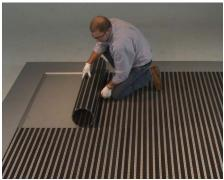
**21** Care & Maintenance: to properly clean underneath the grid and avoid rail damage, roll back the grid edge to the 12th rail. Continue to roll back the grid holding that diameter.
