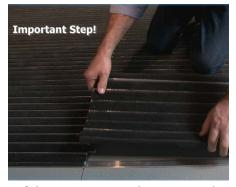
**9** If the section is too long, it may be necessary to tuck the module into the frame to contract the rails.
