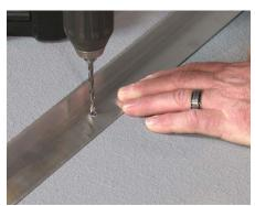
**3** Using the 5/16" masonry bit, drill into the concrete 24" on center. Fasten the frame with the supplied masonry anchors using a #2 Phillips-head screwdriver.
