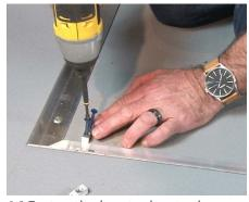
**16** Fasten the locator bar to the floor using the supplied masonry anchors.
