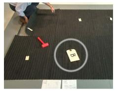
**4** Grid modules are tagged alphabetically in order of placement. Install into the recess accordingly. For odd-shaped layouts, refer to the supplied shop drawings.
