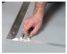
**14** Roll back the mat. Using the recorded dimensions, mark the locations on the concrete, off-set from the frame.
