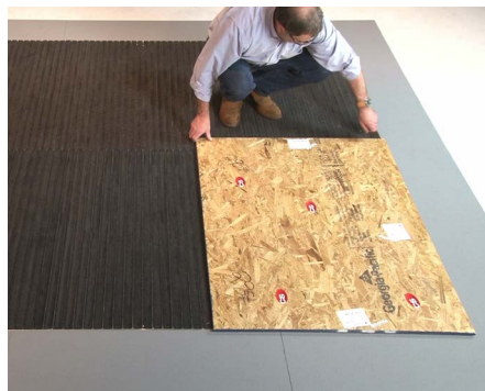
23 Clean the unit with a vacuum. If construction is to continue in the building, protect the unit with plywood sheathing.
