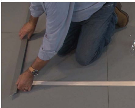
4 Apply the frame to the substrate.
