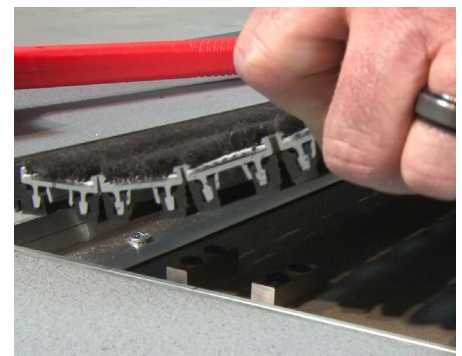
21 Roll the mat forward so that rails fit snug over locator bars to achieve dimensional fit of the unit.
