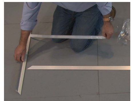
3 Remove the backing from the double-sided tape.
