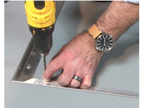
18 Using 5/16" masonry drill bit, drill out both holes for the locator bar anchors to center the supplied locator bars on the lines marked on the floor.
