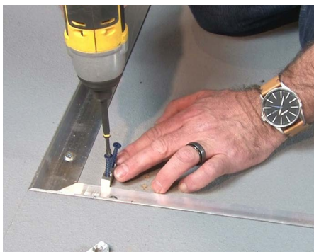
19 Fasten the locator bar to the floor using the supplied masonry anchors.
