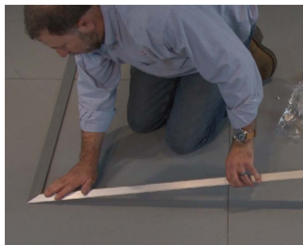
5 Make sure the frame is square and the miters butt properly.
