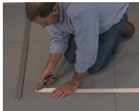
2 Prepare the flooring surface to allow the tape to properly bond to the floor.
