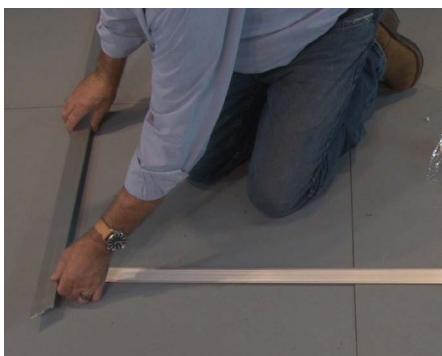
4 Apply the frame to the substrate.
