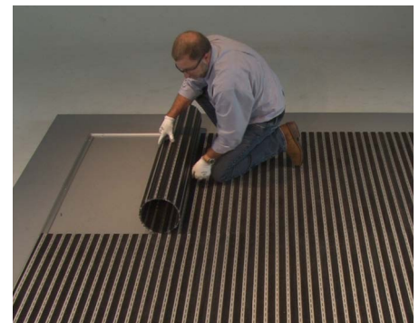
24 Care & Maintenance: to properly clean underneath the grid and avoid rail damage, roll back the grid edge to the 12th rail. Continue to roll back the grid holding that diameter.
