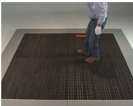
13 Make final adjustments for rail alignment.
