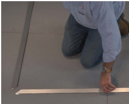
1 Place the pre-mitered tapered aluminum frame at the correct floor location.
