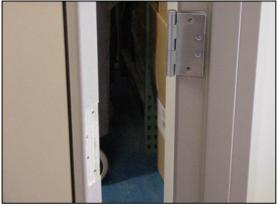
2. The Acrovyn® edge can be removed by inserting something like a flat blade or a screwdriver at the top between the edge and stile and disengaging the return leg from the stile. Once the edge has been removed several feet from the top of the door, strip the remaining portion by pulling it off the door.
