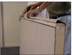
3. If the hardwood stile must also be replaced, unscrew and remove the damaged hardwood stile. Move to STEP 7 if the hardwood stile does not need to be replaced.
