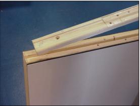
4. The replacement stiles will be pre-drilled and countersunk, ready to be installed. Simply position the stile and secure it to the door. Be careful not to over torque the screws. The new edge can be installed by hooking one leg into the groove between the door and stile and snapping the other leg over the stile and into the groove.
