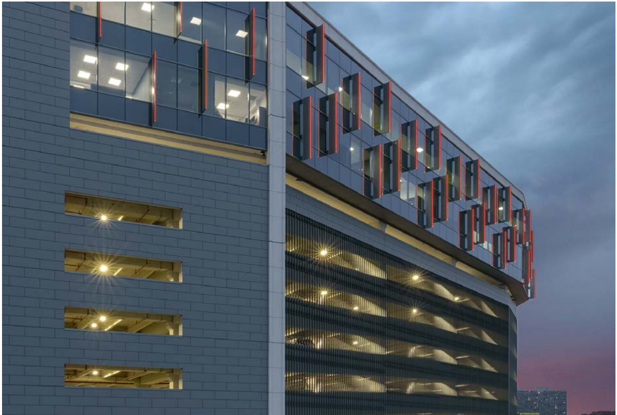
Cablevision Call Center and Parking Garage, Newark, NJ Architect: Rotwein & Blake Photography : David Patino
