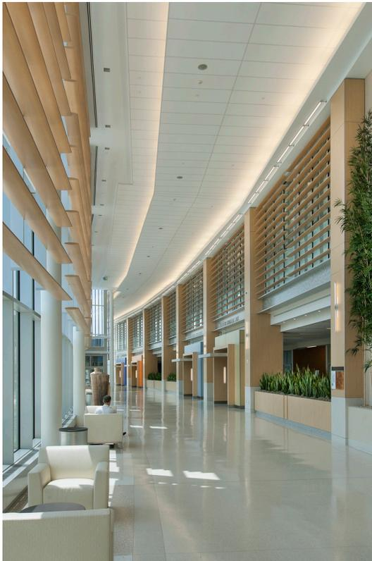
Inside the expansive atrium is filled with natural light from windows that span the length of the building. C/S Wood Wrapped Airfoils, a new interior shade product, are positioned strategically in front of the windows to help regulate and diffuse the sunlight. Used in conjunction with screening attached to the exterior curtain wall reduces the energy required to heat and cool the facility. The same shades are used as an aesthetic feature in other interior areas.
