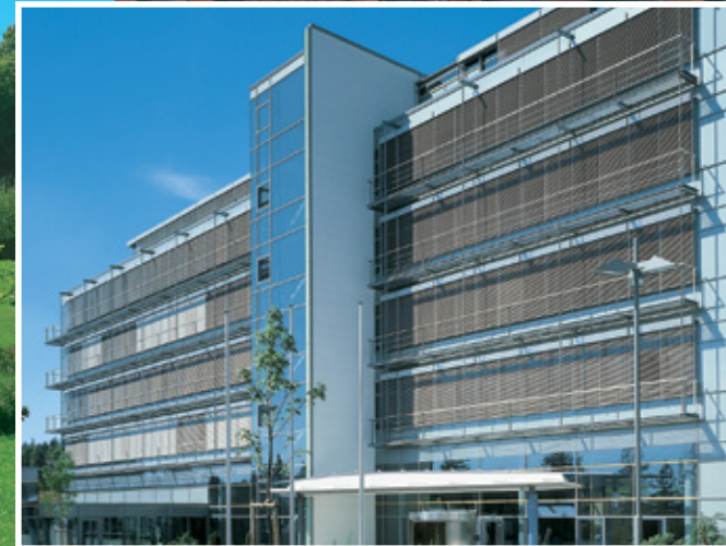
◀ The energy required to cool the curtain wall building, shown at left, was much higher than expected, even with fixed sunshades. The owner added Solarmotion Architectural Blinds and reduced the building's energy consumption by over 30% per year.
