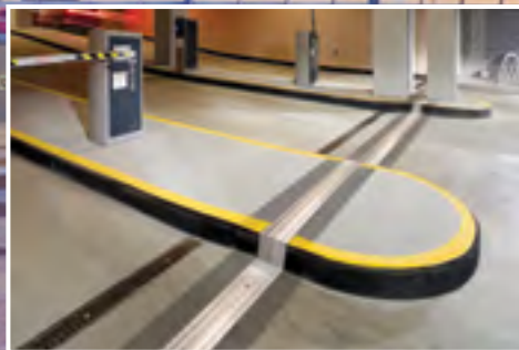
KB Seismic Cover @ NASCAR Hall of Fame
